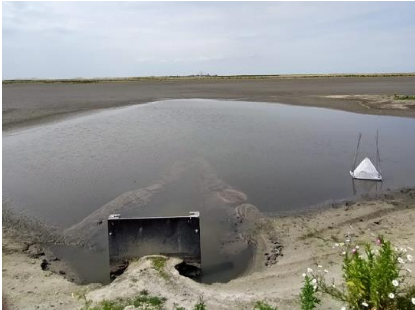
Figure 10: Outlet of inland water at island C, photo from July 2021 when the island was getting drier (Photo made by author)
