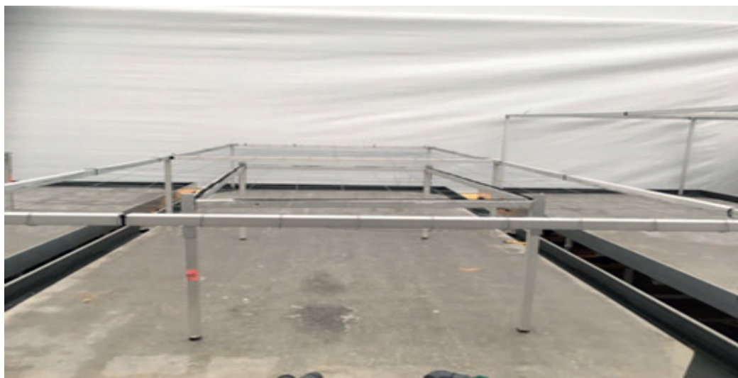
Figure 4 The construction with aluminium frame to support the glass and the surrounding screen to avoid lateral radiation.
