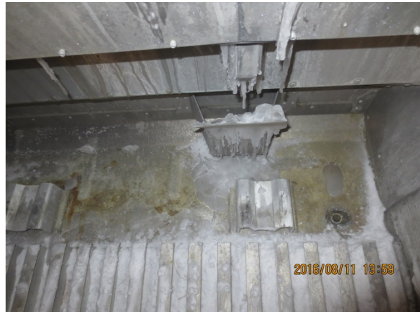
Fig. 26, ice on right-side of floor at end of test 1.
