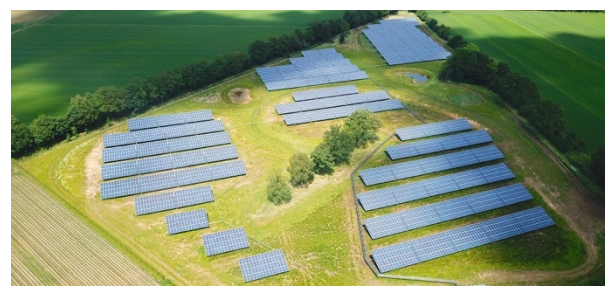
Figure 9 Overview of solar farm Laarberg. Retrieved April 2, 2020 from https://solarmagazine.nl/nieuws-zonne-energie/i16298/greenspread-opent-zonnepark-laarberg-van-2-23-megawattpiek
