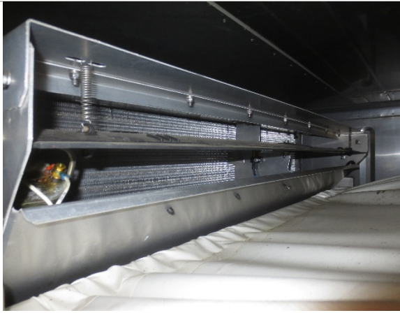
Figure 6 Supply air outlet above air chute.
