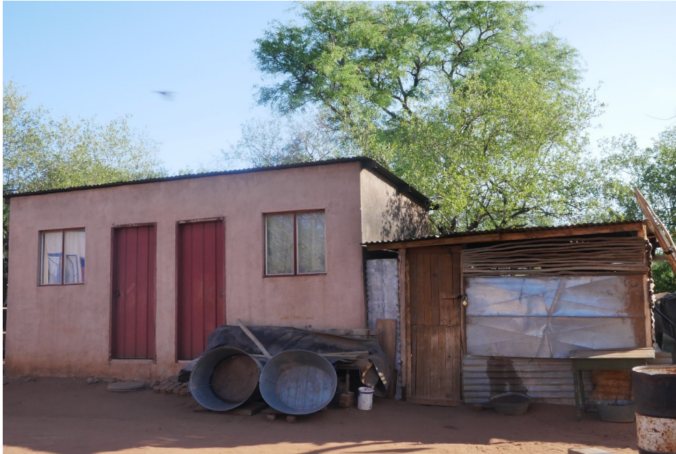
Figure 4.2: One of the four structures that were originally built by Boschpoort Ondernemings (Pty) Ltd. (picture by the first author, 2019).
