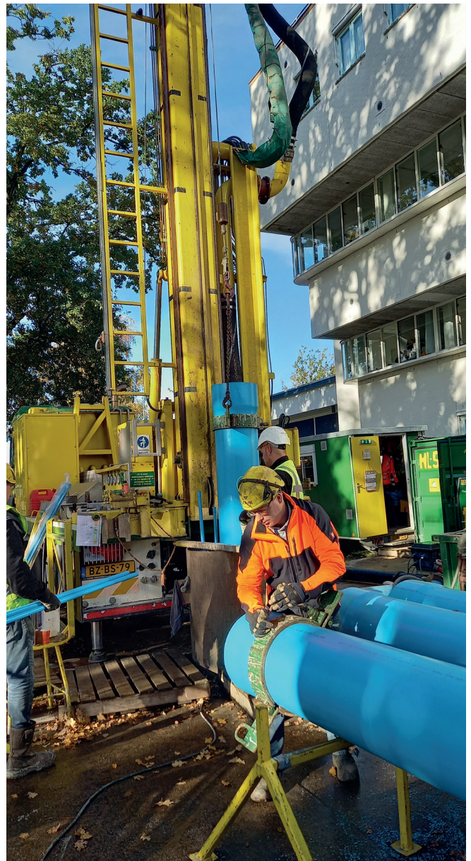
Fig. 6: We stick the tubes and filter tubes together and lower them into the shaft along with sampling tubes.
