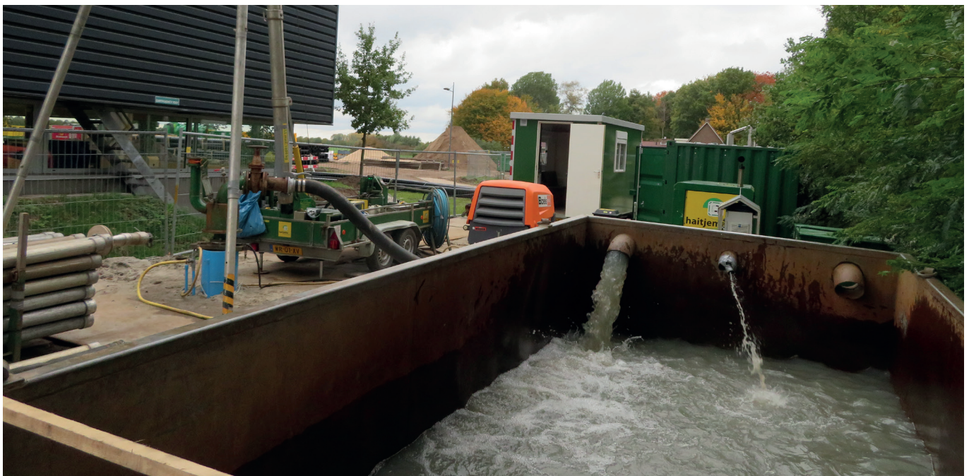
Fig. 9: The pumped-up water is monitored to see whether the well is clean.
