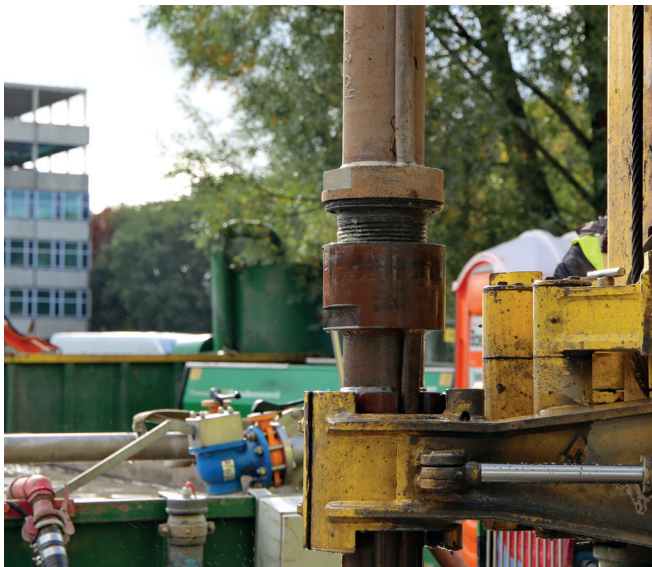
Fig. 3: Drilling rods are connected together.
