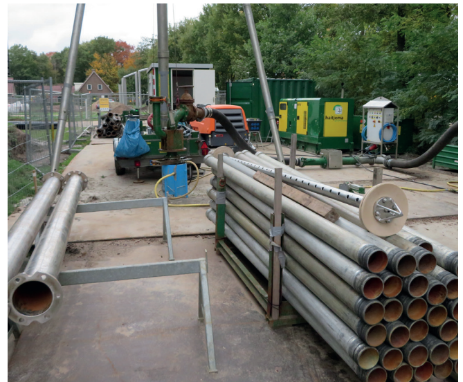
Fig. 8: Equipment for developing the well, with the sectioning device at the front.
