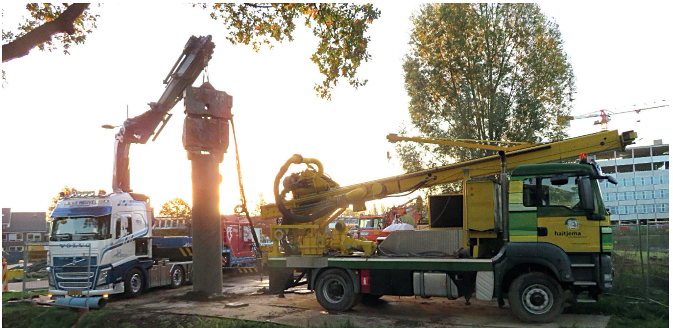
Fig. 1: The conduit is vibrated in.
