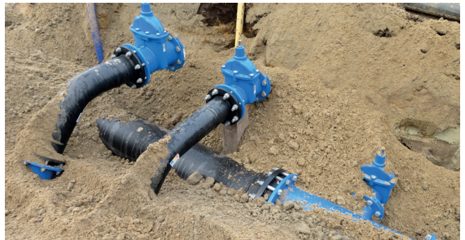
Fig. 9: Branches with valves have already been installed for future connections. Everything is in position, so the trench can be filled in.
