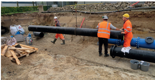
Fig. 3: Using the crane, the pipework is brought to the right place.
