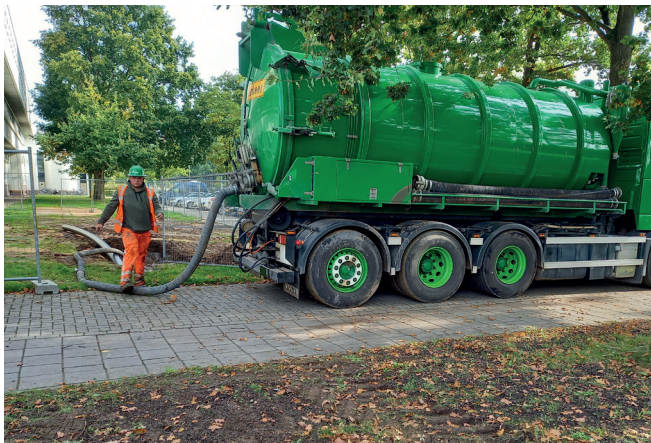
Fig. 7: "Done! The remaining bentonite-sand mixture is sucked out and disposed of."
