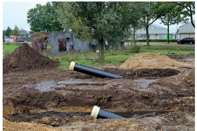
Fig. 8: Two pipe ends on the surface ready to be connected.
