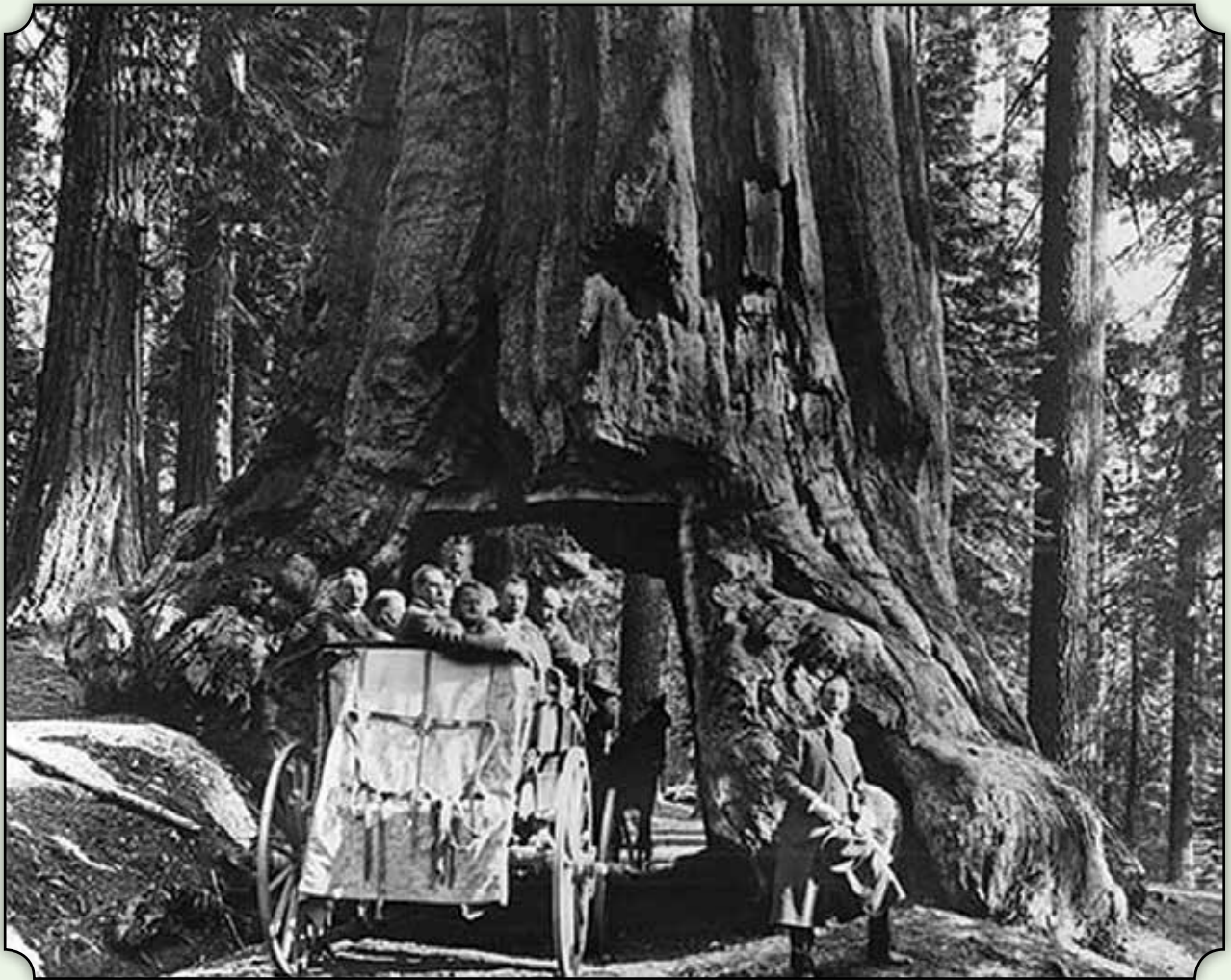
Foto: Harpers Ferry, National Park Service Historic Photograph Collection
