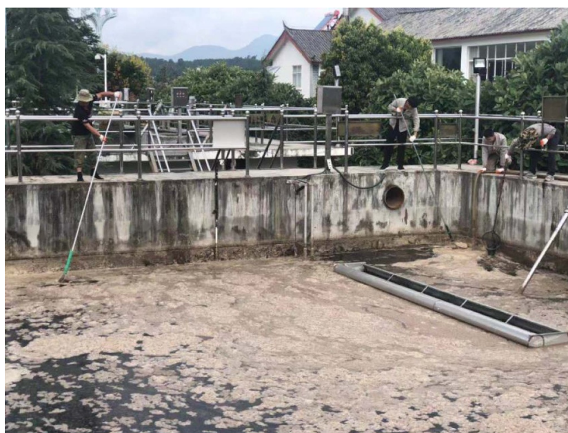
Figure 4. Floating oil and fat from kitchen wastes on the oxidation pond of a sewage treatment plant in Lijiang city, a tourism hot-spot in south China, following the implementation of the ASF control policy in 2019, which prohibited swill feeding to pigs. The table presents the mean total nitrogen (TN) concentration of the water in the adjacent river, which receives the effluents from the treatment plant, in 2017 and 2019.
