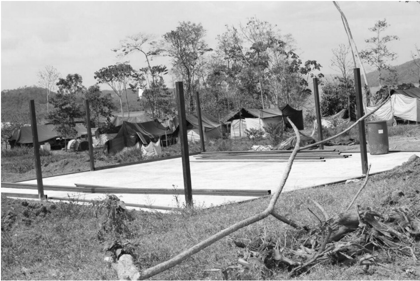
FIGURE 3.3 Lack of infrastructure in Gallo. Courtesy of Maria Quiroz
