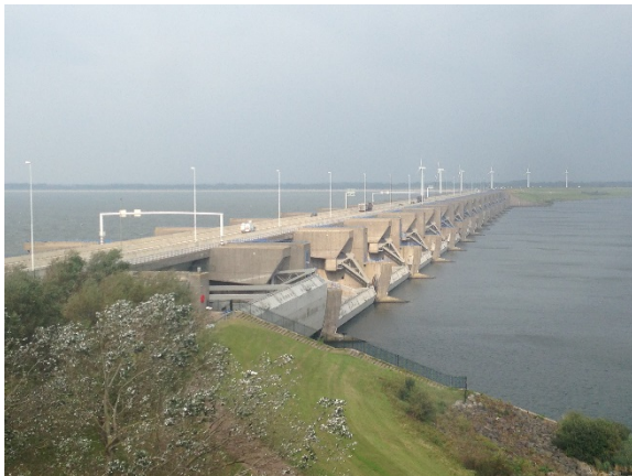
Figure 14 – Haringvliet sluices, the storm surge barrier between the mouth of the Rhine and the North Sea.
