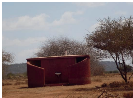
Figure 5.1: A sanitation facility at Osiram Women cultural Boma Source: Authors.
