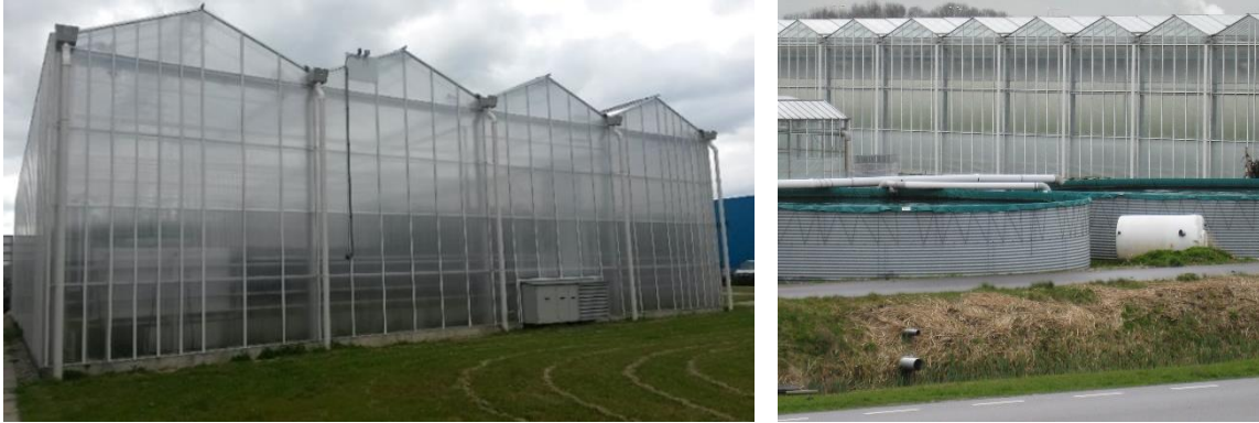
Figure 2. High-Tech greenhouse (Wageningen University and Research facility in Bleiswijk, NL), characterized as houses with diffuse glass, with a gutter height of 7 m, rainwater collection (left) and rainwater collection tanks and drainage pipes to the ditch (right).
