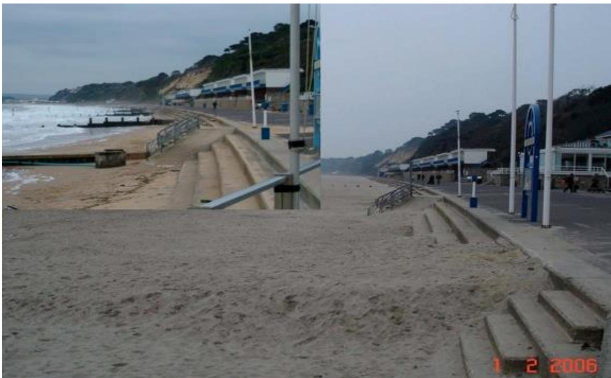
*Figure 3. Before and after: beach nourishment using dredged sediment from the deepening of the navigation channel in Poole Harbor*
