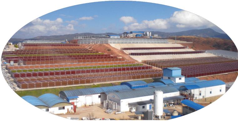
Fig. 7-4 Yunnan Alphy Biotech Co, a tubular photobioreactor plant, China ( Haematococcus ). Photograph: Courtesy of prof. Liu.
