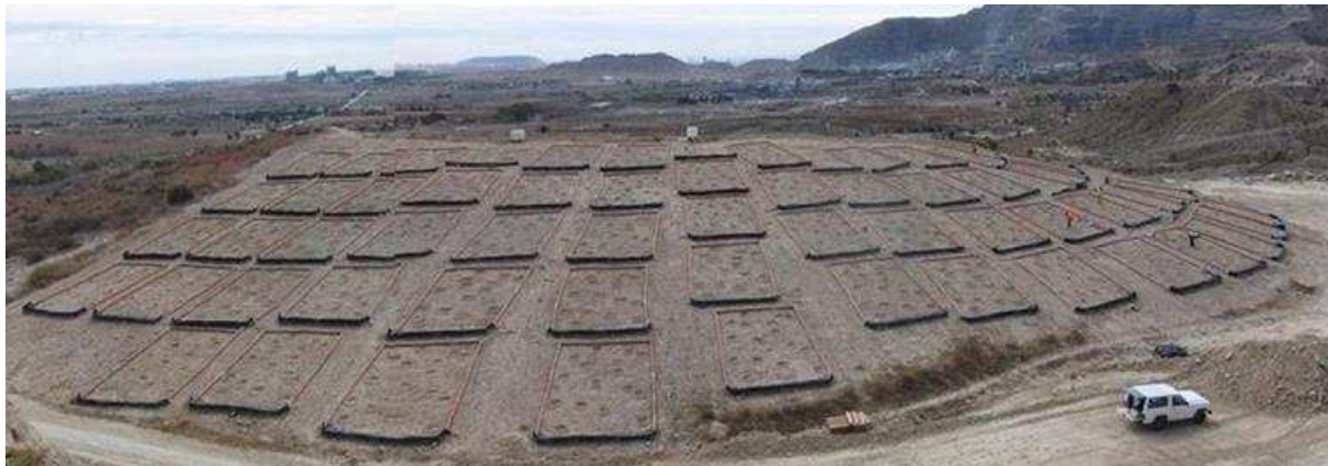
Figure 3. General view of the experimental station ES56 in Alicante (Spain) on an artificial slope with degraded soils built ad hoc for experimental purposes. Photo by S. Bautista.
