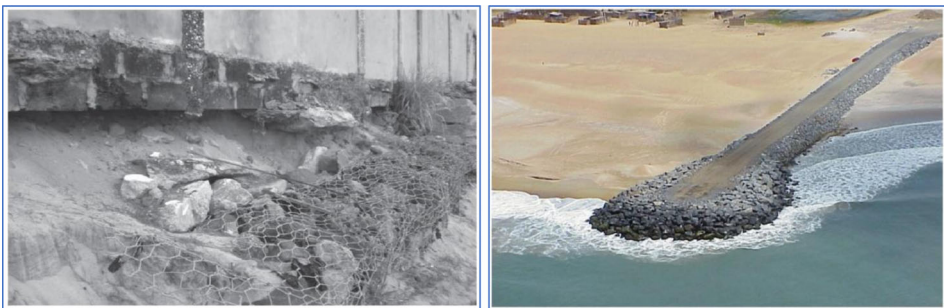
Figure 3. Passive adaptation (left): using rocks in human settlements on the Benin coast (Dossou and Gléhouenou-Dossou 2007). Active adaptation (right): groins along Keta in Ghana (Angnuureng, Appeaning Addo, and Wiafe 2013).
