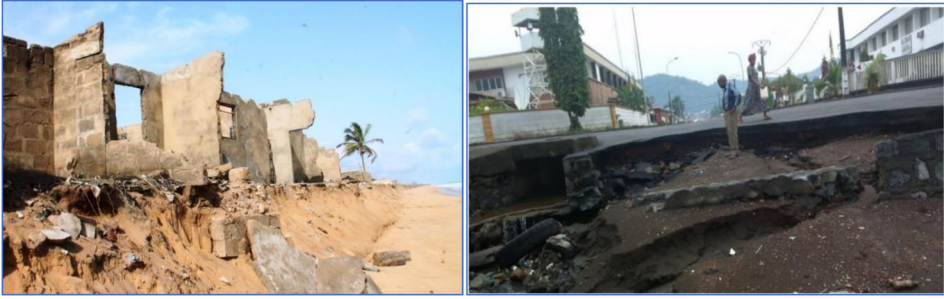
Figure 2. Right: Disappearing buildings in Aneho, Togo (Addeh 2015). Left: Marine Erosion of the coastal highway in Limbe, Cameroon (Kometa et al. 2016).
