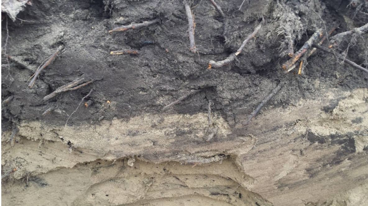
Figure 4 Rootstocks of Asian knotweed in the dark covering layer of the rail embankment at Kop Weespertrekvaart, Amsterdam.
