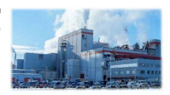
Licella. The proposed plant will use Licella's Cat-HTR<sup>™</sup> technology to convert residues from the pulp and paper factory into Hydrothermal Liquefaction (HTL) bio-crude at a rate of 500 000 barrels per year. A CAD 13M grant from Sustainable Development Technology Canada was awarded in March 2017, towards the CAD 39M project.
