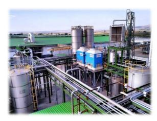
Energy acquired the international intellectual property rights for the CatLiq® technology in 2011. The demonstration plant was built by Altaca Energy based on the SCF Technologies pilot plant, which was relocated to Gebze, Turkey. The plant converts various biomass sources, including biogas plant digestate, forest waste, sewage sludge, agricultural waste, food plant waste, organic household waste, into a HTL bio-crude, with 70% recovery of process heat.
