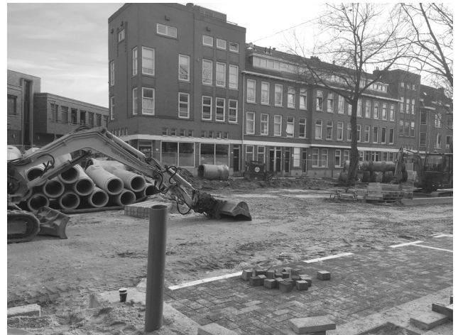
Fig. 4.2 Polderbaan broken open and redesigned to renew the sewer
