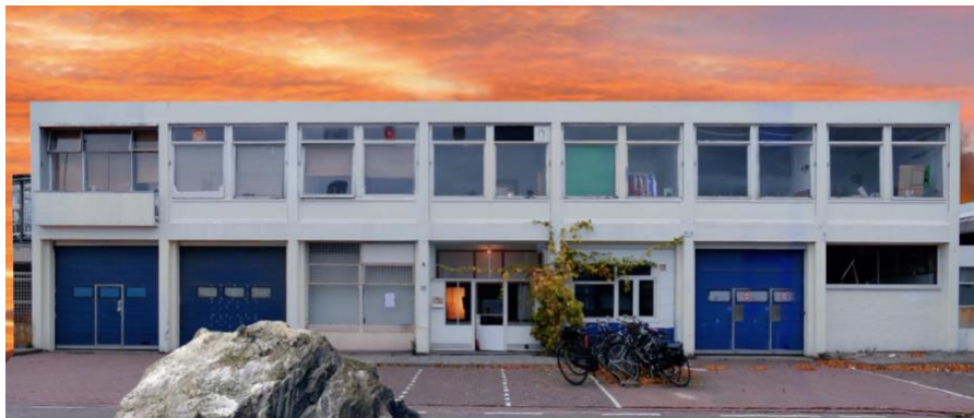
Figure 19: Facade of ISO Amsterdam in Sloterdijk. Source: (ISO Amsterdam, n.d.).
