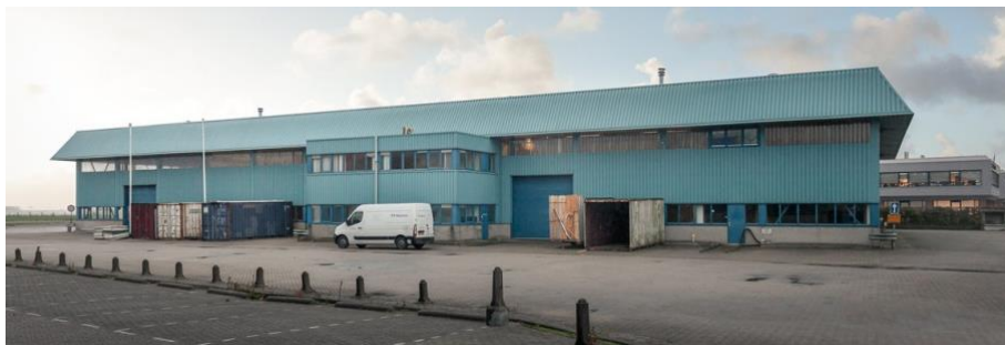
Figure 15: Facade of the Workplace in Bogota. Source: (Breeding Place Bogota, n.d.).
