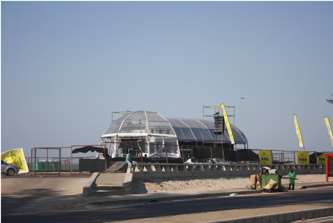
The temporary enclosure of one of the parking lots lining the Marginal, for a private event sponsored by Savanna (a South African cider company). These exclusive, temporary clubs have capitalised on the Mozambican tradition of beach-side partying, but turned it into an increasingly high end affair.
