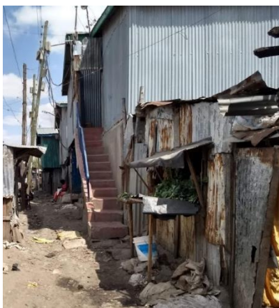
Figure 4 Combined residential and commercial land use in Lunga
