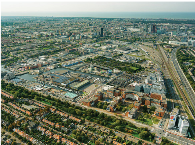
Figure 5.3 Aerial picture that demonstrates the Binckhorst’s diversity a
