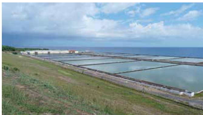
Yaguanabo Shrimp hatchery with ponds for broodstock in front and in-door facilities for reproduction, larvae rearing and algae rearing at the back
