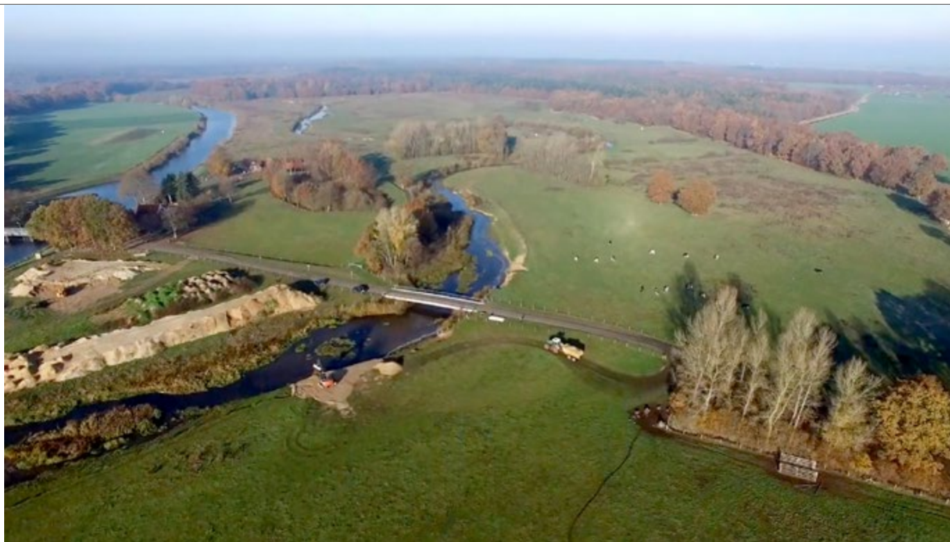
Sand replenishment on a side arm of the Vecht River in Overijssel province. The aim is that the river itself deposits sand so that the riverbed is raised, the flow is slowed down and the water level goes up.
