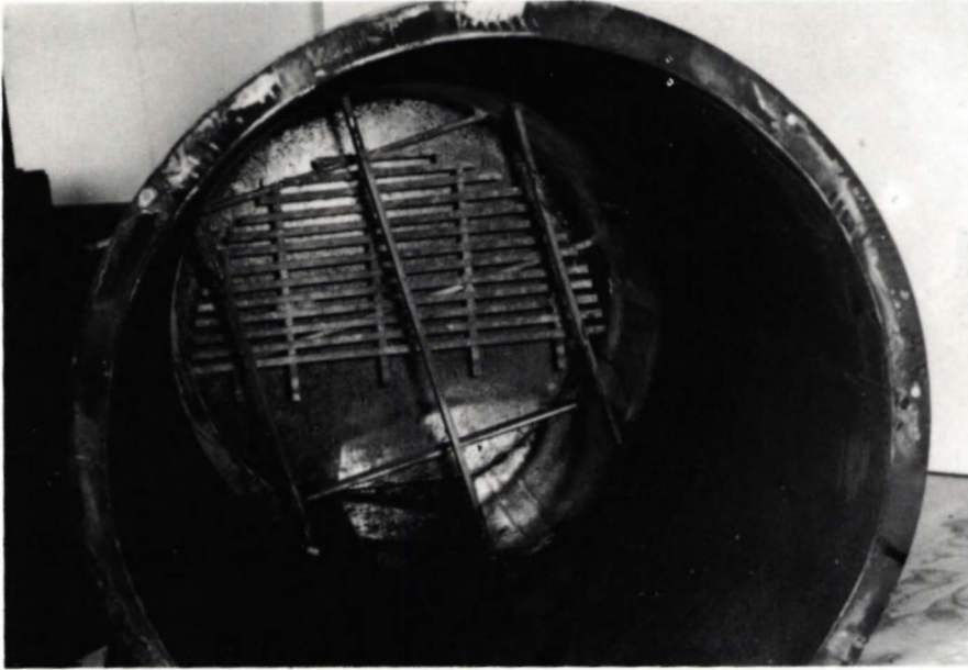
Fig.12 Top inside view on the stays for the steam drum and the fire grate.
