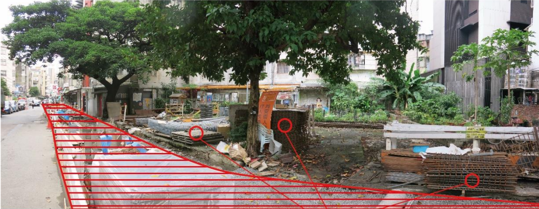
Pedestrian pavement project is running
