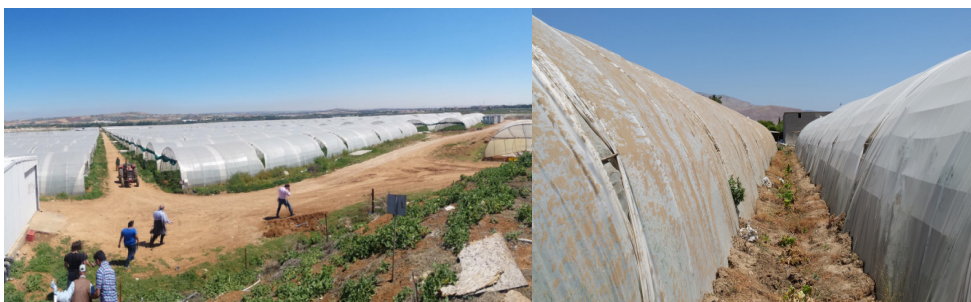
Figure 1. Typical Jordanian single tunnel greenhouse with small slits for ventilation and mud over the roof for shading.
