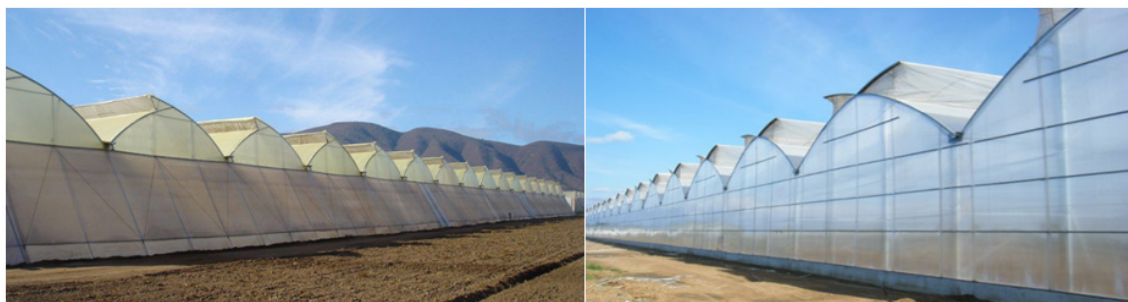
Figure 2. The two types of greenhouse structures simulated: multi span greenhouse with a single fixed roof vents (left); multi span greenhouse with double automated roof vent on each span (right).
