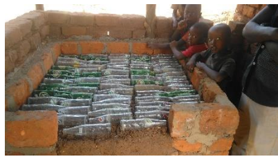
Figure 25 Isolating the oven floor
