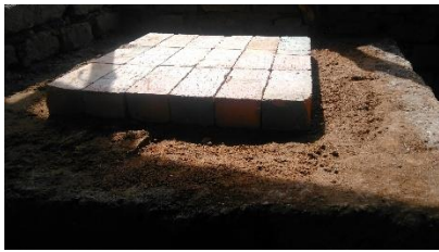
Figure 28 Laying refractory bricks
