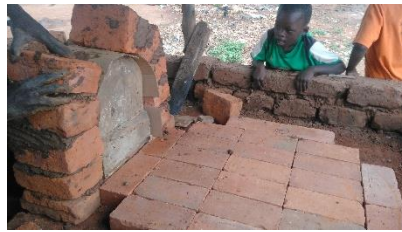
Figure 27 Building oven door
