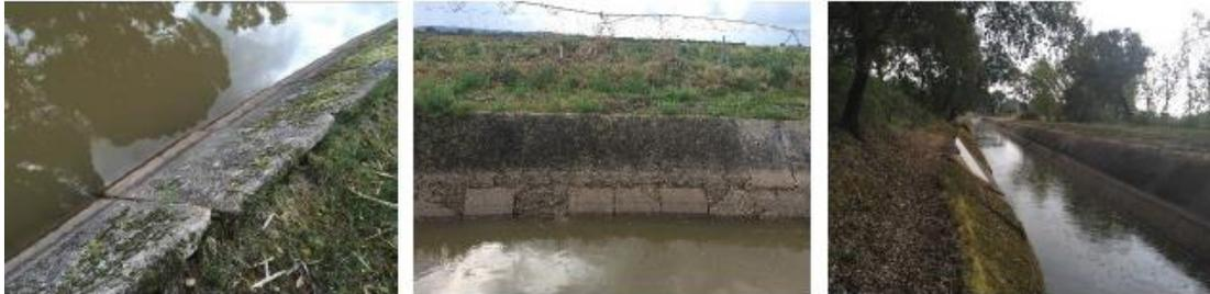
**Figure 5.12: Canal walls deterioration**
