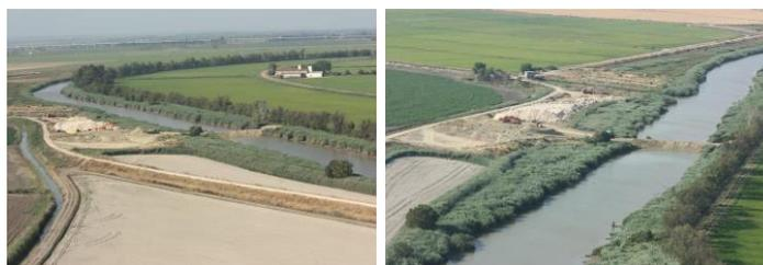
**Figure 6.16: Temporary weir in the Sorraia river during the 2012 drought (July 2012, source: ABLGVFX).**
