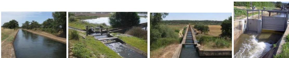
**Figure 6.12: Sorraia valley PIP. Water distribution (channels and floodgates)**
