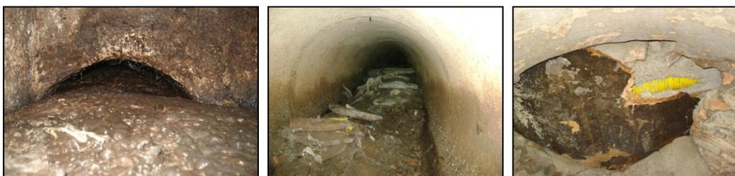
**Figure 8.3: Sedimentation and structural problem in the Badalona sewer network.**
