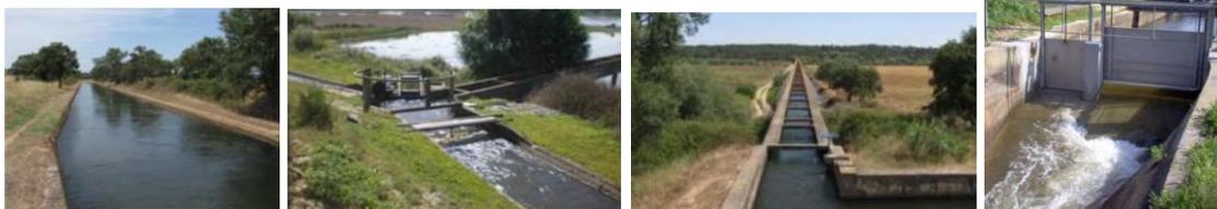
**Figure 6.12: Sorraia valley PIP. Water distribution (channels and floodgates)**
