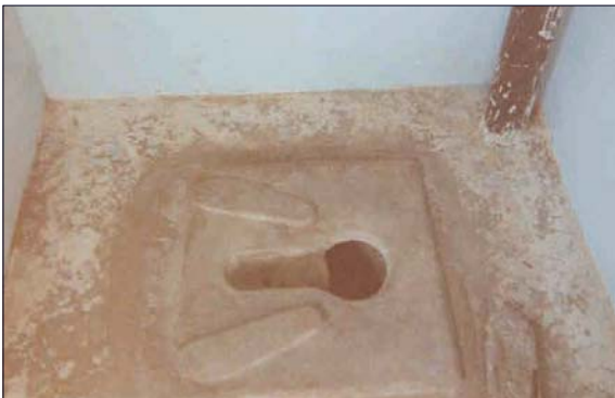
Figure 8 - Anaerobic treatment of black waste(water) in Tanzania, family.
