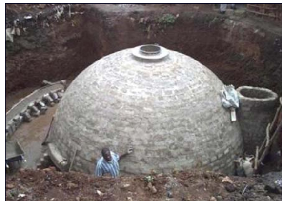
Figure 14 - The SPARC-style sanitation block in Gatwera village in Kibera, Nairobi.
