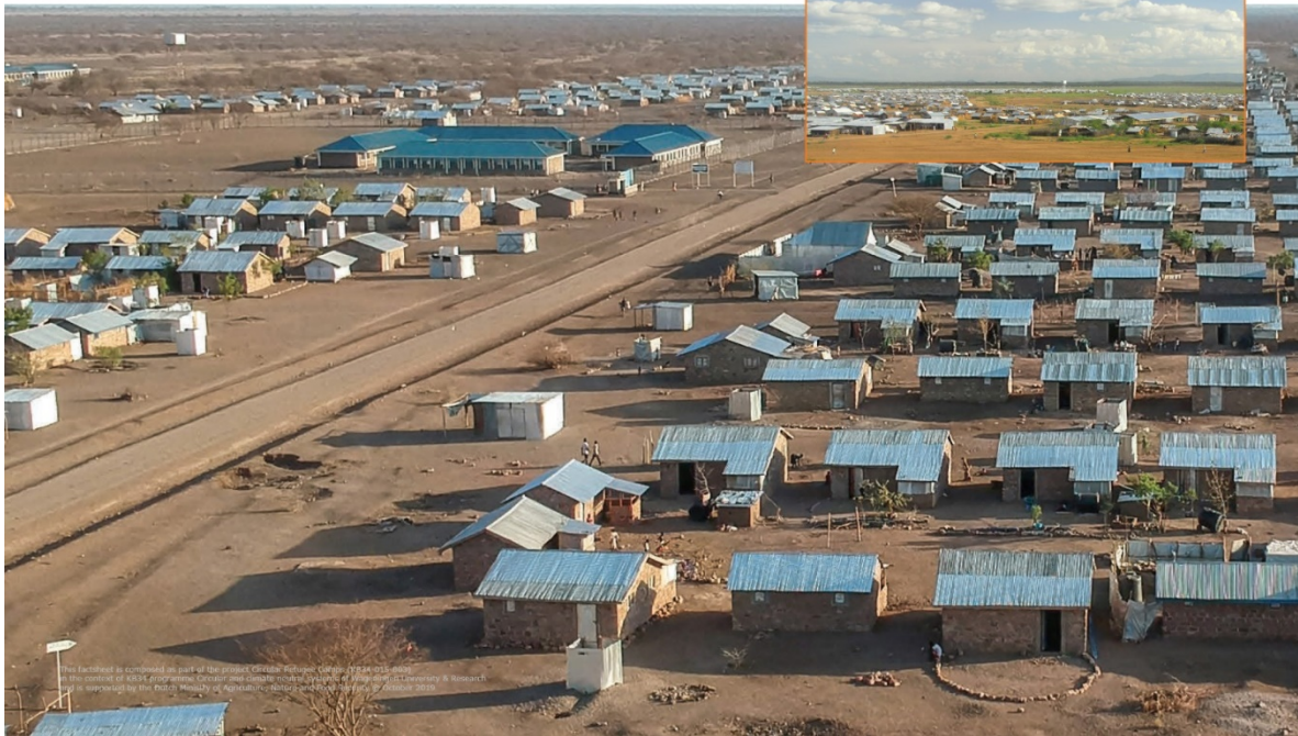
An aerial image of the over 2,000 permanent shelter units constructed in Village One of Kalobeyei Integrated Settlement. UNHCR/Samuel Otieno
