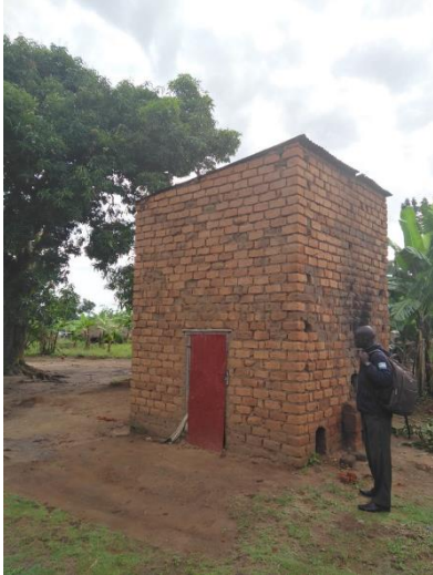
Tobacco curing facility.
