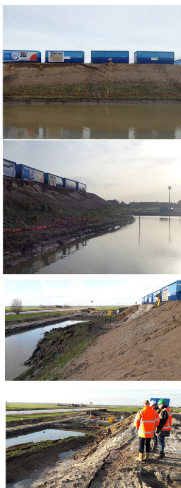
Figure E.1: Photographic report of the Green dyke failure
