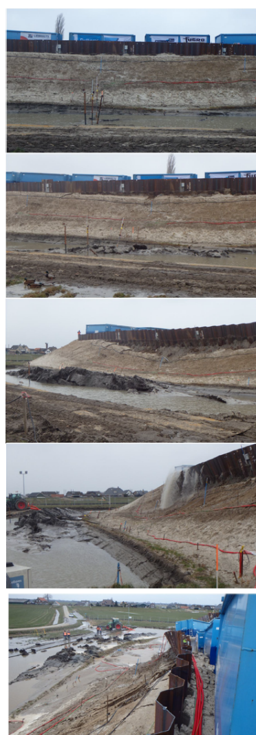
Figure E.2: Photographic report of the Blue dyke failure
