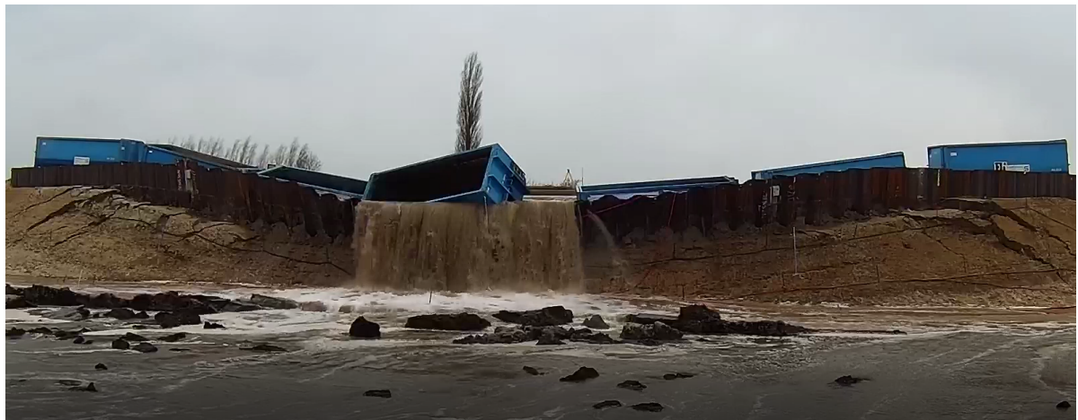
Figure 1.1: Picture of the failed dyke with sheet pile wall
