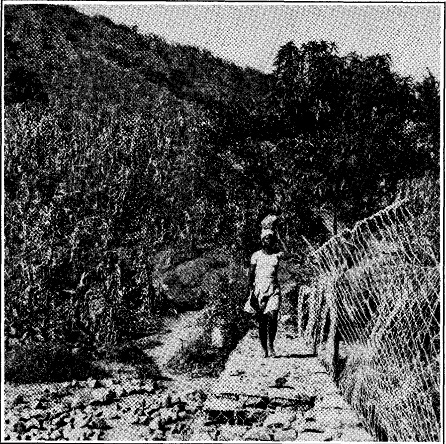
Women are contracted to carry material like building stones.
