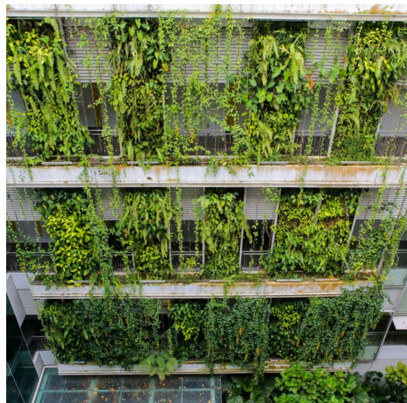
Figure 13: Incorrect application of vertical greenery. Tan (interview) explains that there are two failures here: the system is not accessible to maintenance and the hybrid between an LWS and support system will never be successful since they overgrow each other. Source: http://www.fas.nus.edu.sg/srn/archives/photos-bank/gr
