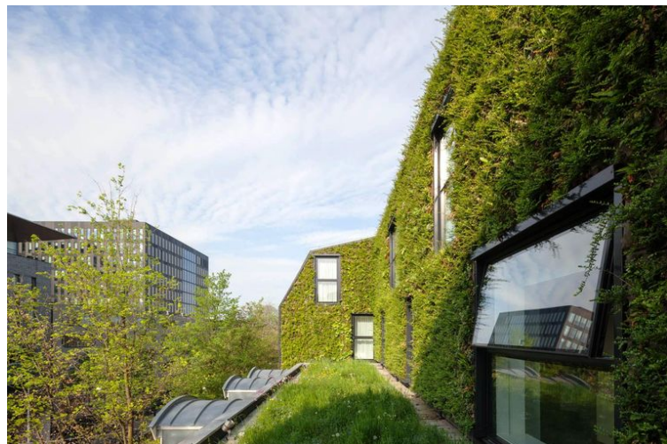
Figure 17: An example of professional application of vertical greenery at the Hyatt Regency in Amsterdam by Sempergreen. Source: Sempergreen.
