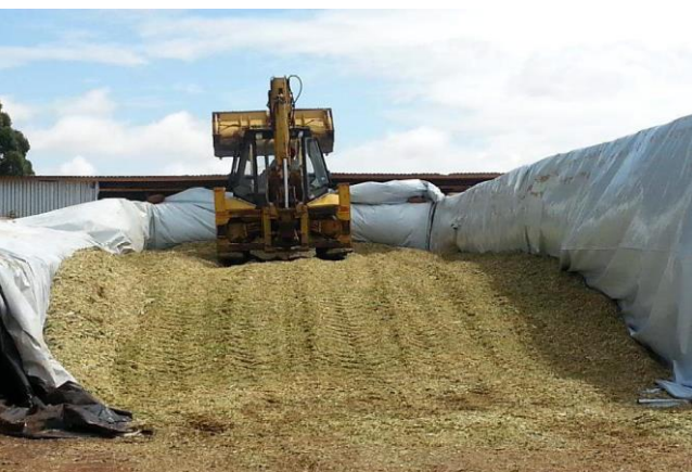
Contractor making the silage bunker
