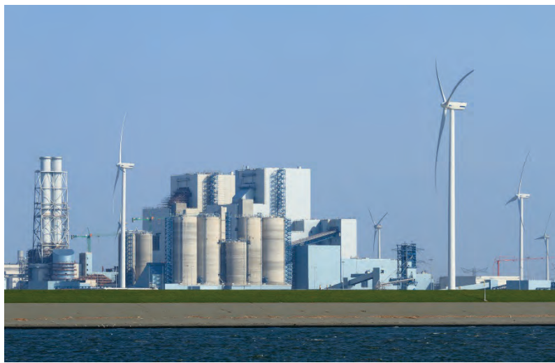
Figure 19. Biomass is co-fired in several coal-fired power stations.
