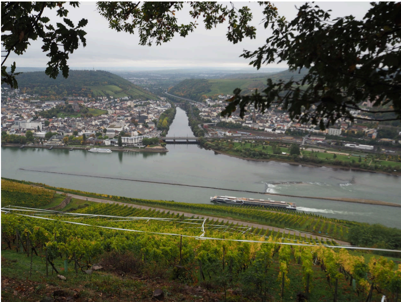
FIGURE 6.2: A longitudinal training dam with both channels of comparable width in the Rhine River near the city of Rudesheim (Germany), October 2017.
