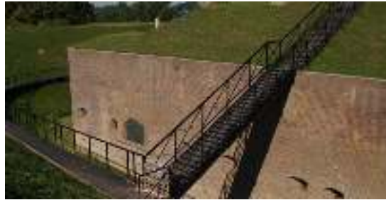
Figure 29: steely handrail of the bridge, source: www.mansveldermetaal.nl
