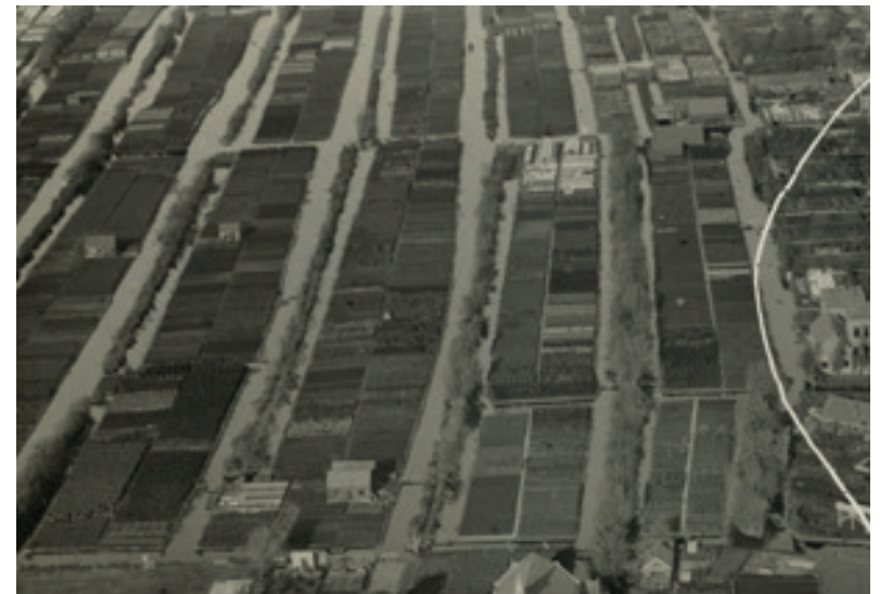
Figure 3.5.3 Aerial picture of houtakkers (FTDL, 1920-1940).
