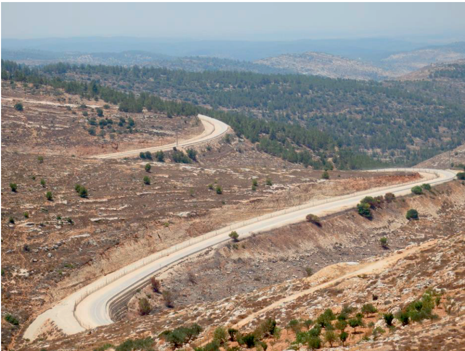
Figure P.3: A section of The Wall north of Ramallah made up of a 4.5 metre high electric fence with a security zone (source: Rijke, July 2016).
