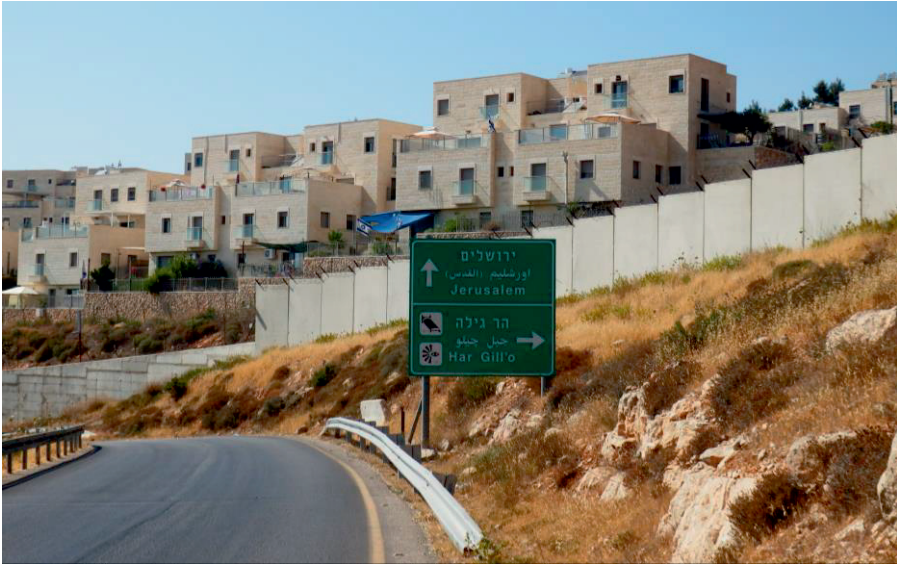
Figure P.5: Har Gilo (source: Rijke, June 2017).
