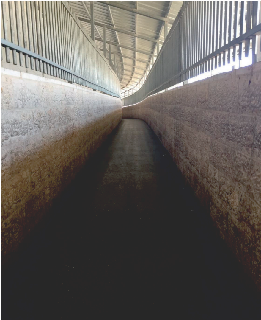
Figure 4.2: The general entry tunnel of Checkpoint 300 (source: Rijke, May 2017).
