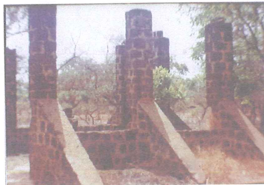
Plate 5. Pillar remains of the defunct Nyange settlement built by the Gonjas with plinthite blocks near Sawla (Northern Region) between 1932 and 1935 as the Yabun-Wura Court during the reign of Yabun-Wura Mahama.
