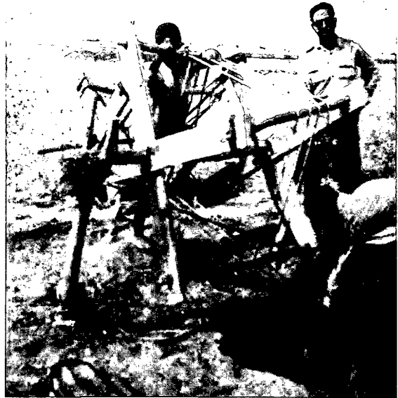
FIGURE 30. Digging ghanats at Chabankareh, South Fars. The dug-out material is put around the "well" and appears as a ring on the aerial photograph (see Fig. 19).
