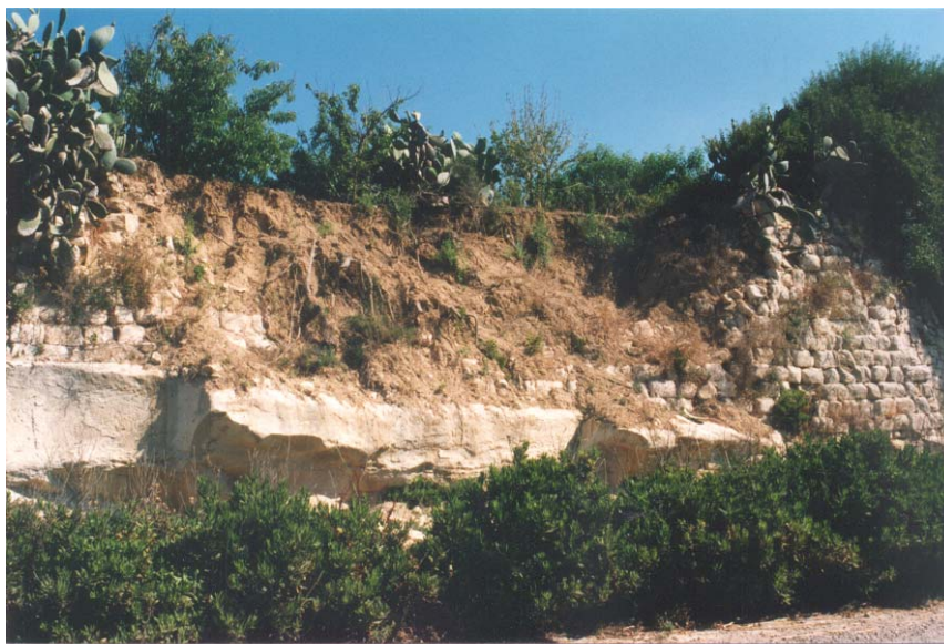
Photo 2. Even the existing regulation prevents demolishing or endangering the rubble walls increased soil erosion brings to their structural damage
