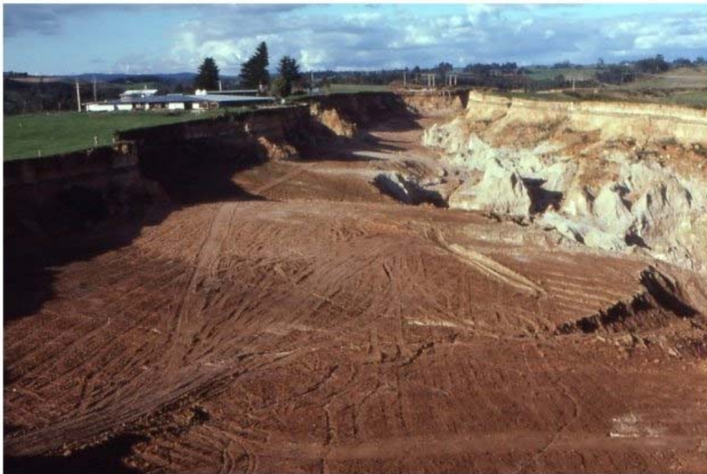
Figure 2. The chasm remaining from when a canal for a new hydroelectric scheme at Ruahihi, Bay of Plenty, New Zealand collapsed in 1981. The failure occurred within sensitive volcanic ashes, forming a flash flood in the adjoining valley (to the right).
